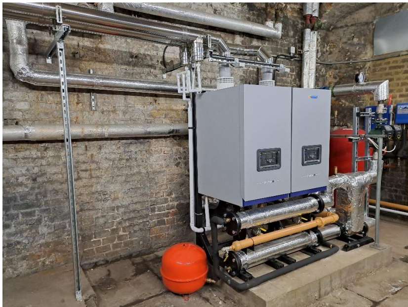
St Dunstan in the West: two new energy efficient condensing boilers were installed in the church's crypt.
