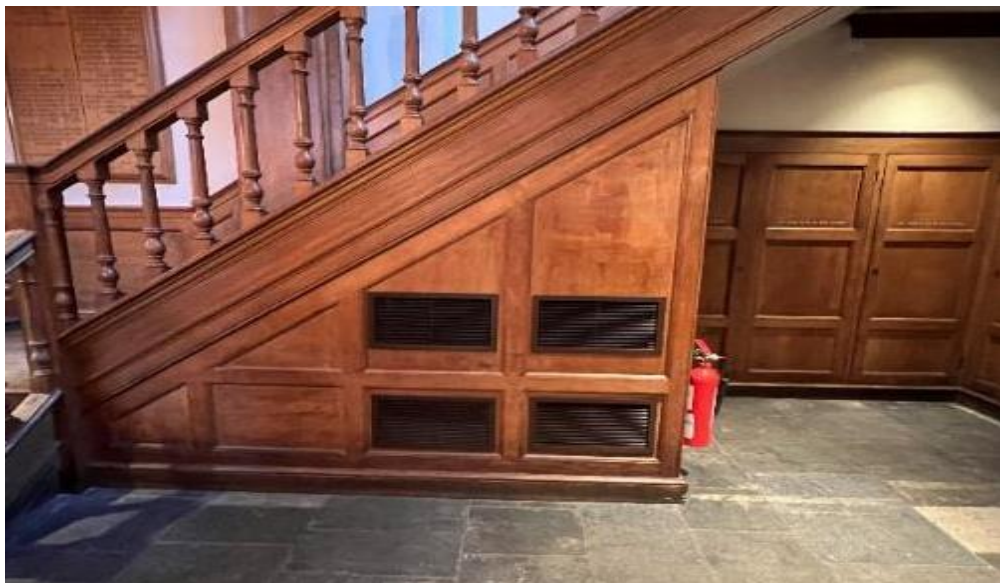
St Andrew by the Wardrobe: heat emitters served by air source heat pumps pictured below
