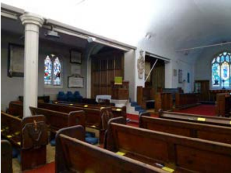
Existing view of the organ chamber from the south west of the nave.
