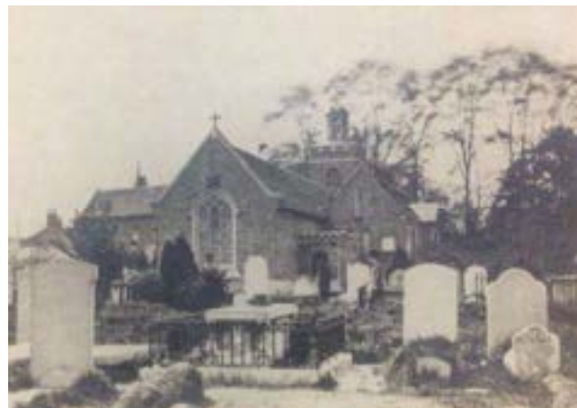
1860: Chancel extended east and robing room to the north.
