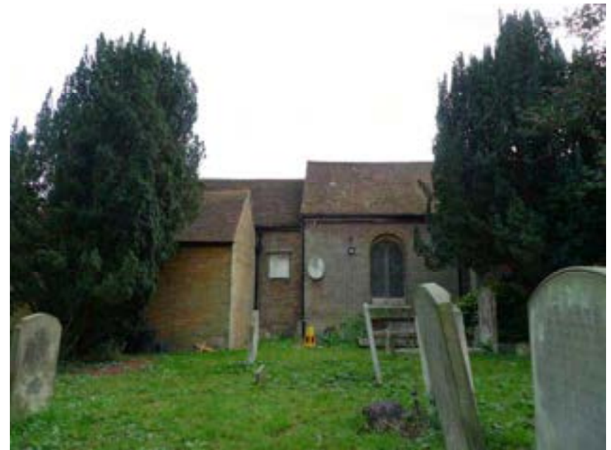
External view of the east window to the north nave aisle
