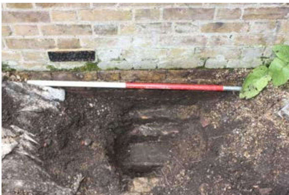
Plate 3: Southwest Facing Section, Test Pit 3, showing foundations
