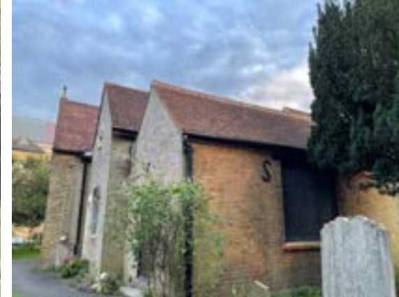
Northeast corner of proposed site.
