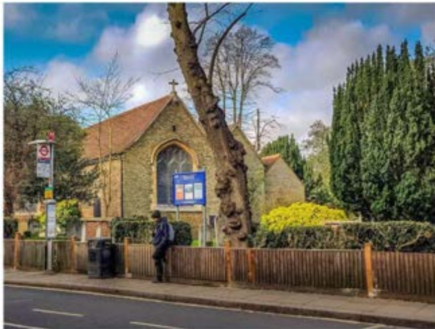
Key view 2: view of the south-west along A313 towards Teddington High Street. The church appears to be nested in the churchyard.
