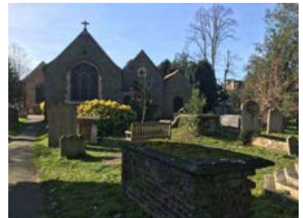
Today (2020) : by 1884 the Organ chamber and clergy vestry have replaced the robing room new choir vestry to the north.
