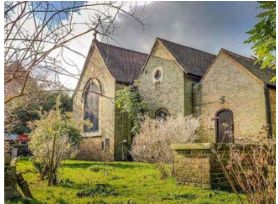
Key view 5: view towards east end of the church from the churchyard.
