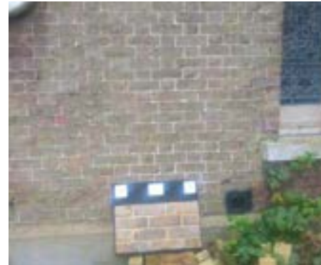
Custom blend sample panel on North elevation
