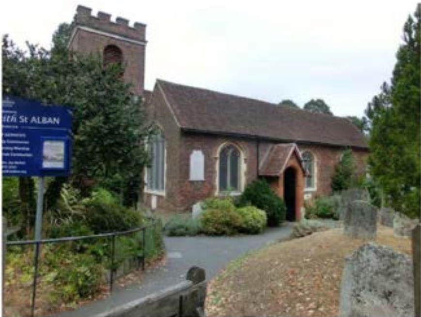
Key view 6: view of the south aisle wall and the first view of the church upon entering from the entrance at the corner of Ferry and Twickenham Road.
