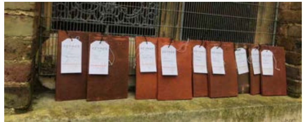
Samples of Keymer roof tiles viewed insitu.
