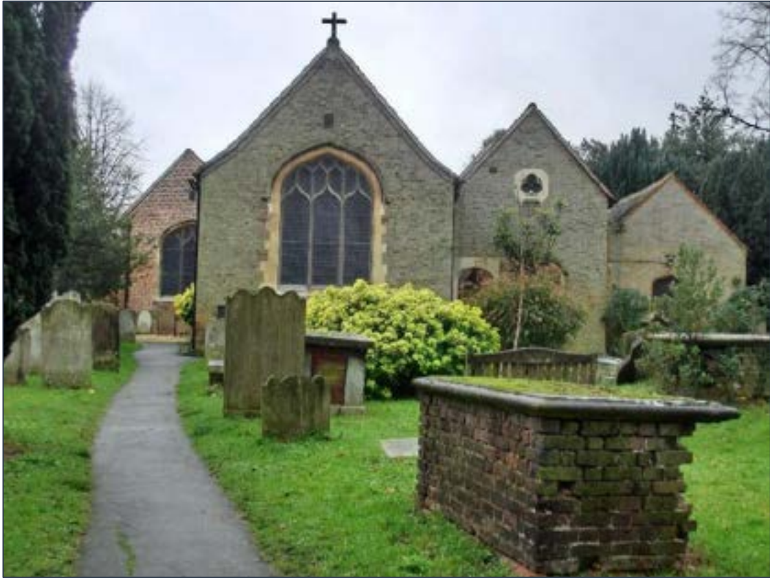
Fig 3. St Mary with St Alban: east elevation viewed from the churchyard path
