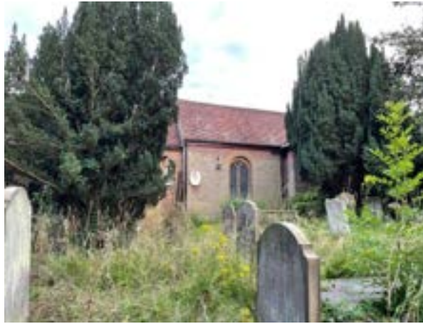
Northern elevation of church
