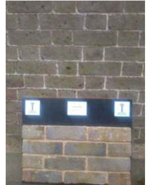
Custom blend sample insitu against east elevation
