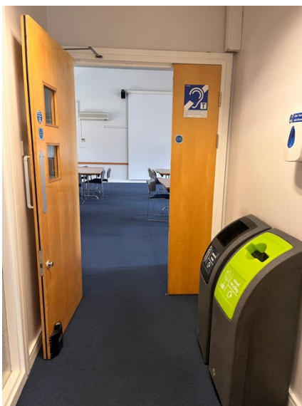
Door to conference room
