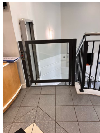
Platform lift goes up to reception
