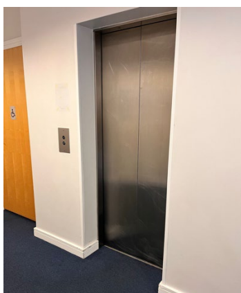
Accessible toilets are by the lifts
